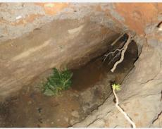
Photos taken above and inside a cavity that has formed on the outside of the Western Service Stormwater Channel due to underground soil erosion. Eventually the cavity will reach a size where it can no longer support itself and will collapse.
