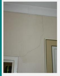
Re-entrant cracks at windows and door frame corners
